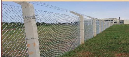
PART OF THE LANDSLIDE/AIRSIDE DEMARKATION FENCE
