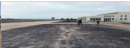
COMPLETED TERMINAL BUILDING AND ONGOING WORKS ON APRON PHASE 2
