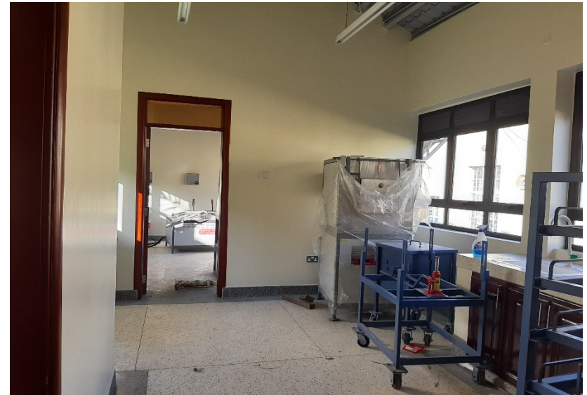
Cupellation furnace in Fire Assay Unit
